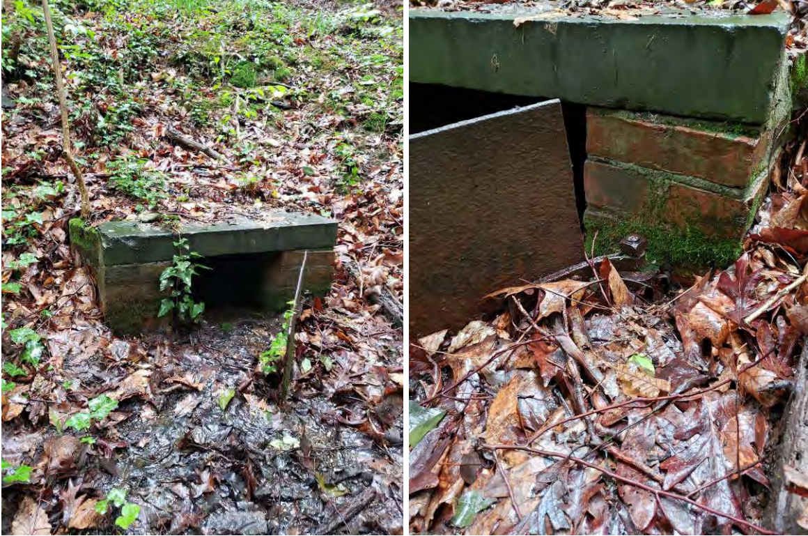
Figure 7-9. Looking southwest at a brick and concrete Spring Box (Feature 1) located within the southern portion of the LOD.
