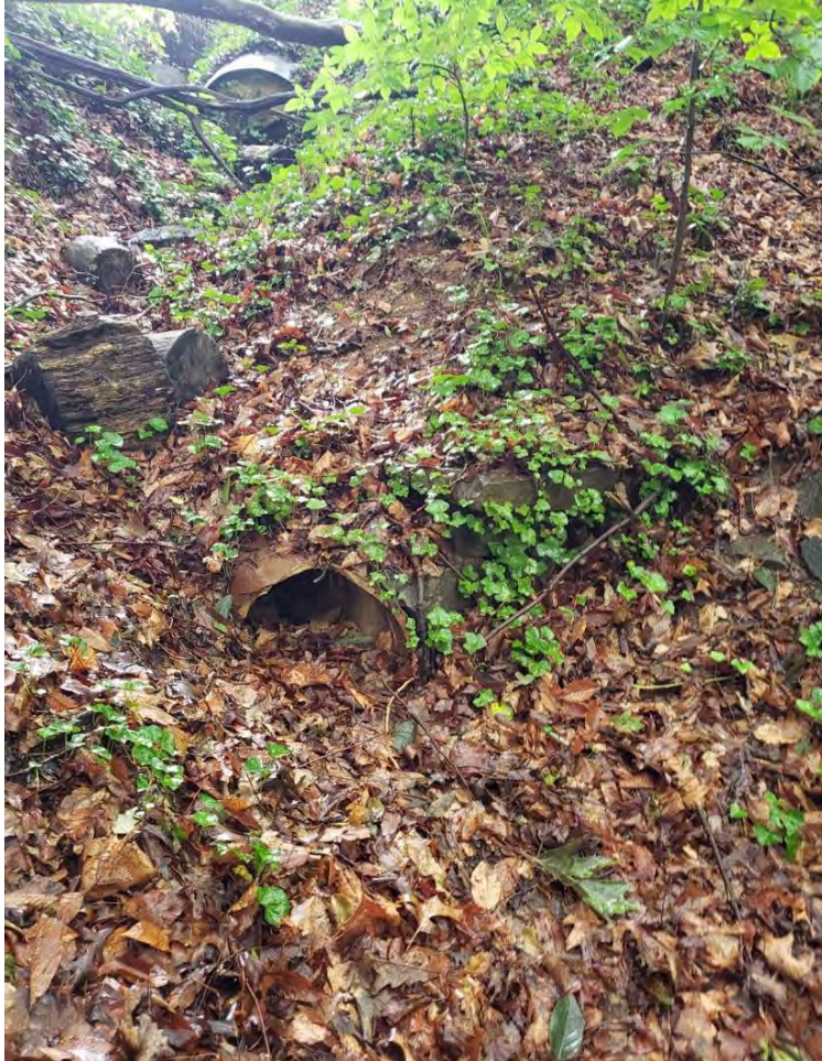
Figure 6-10. View of ceramic drain and riprap (Feature 2) along southern slope below Youth Garden, facing north.
