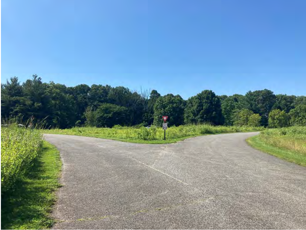
Figure 7-2. Looking south along Ellipse Road, NE towards its intersection with Azalea Road, NE.
